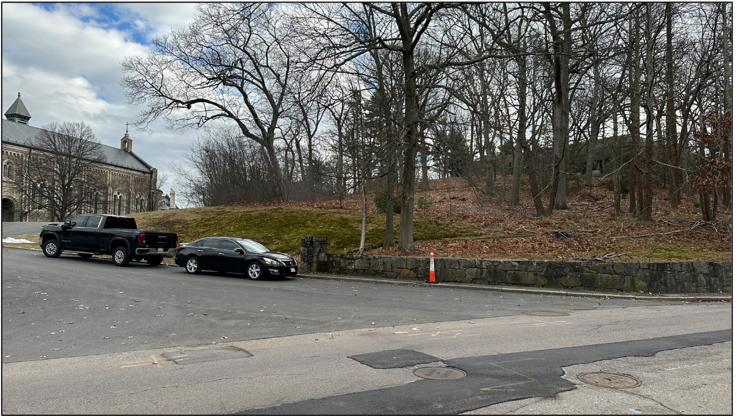
Photograph 1: View of the Project Site from Lake Street by St. John's Seminary's entrance
